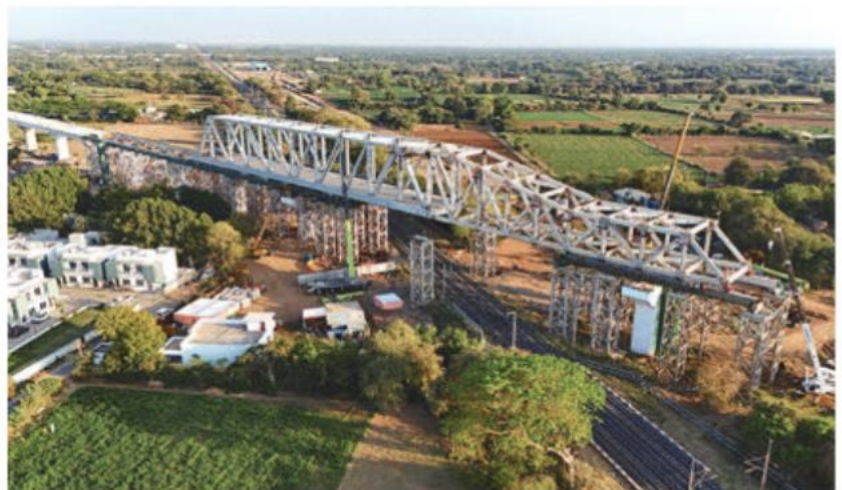
100 m long "Make in India" steel bridge launched at Nadiad, Gujarat
