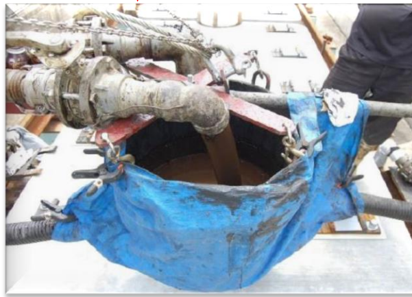
CAM injection for under track slab
