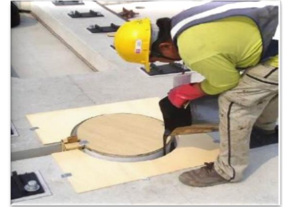
CAM injection for under track slab
