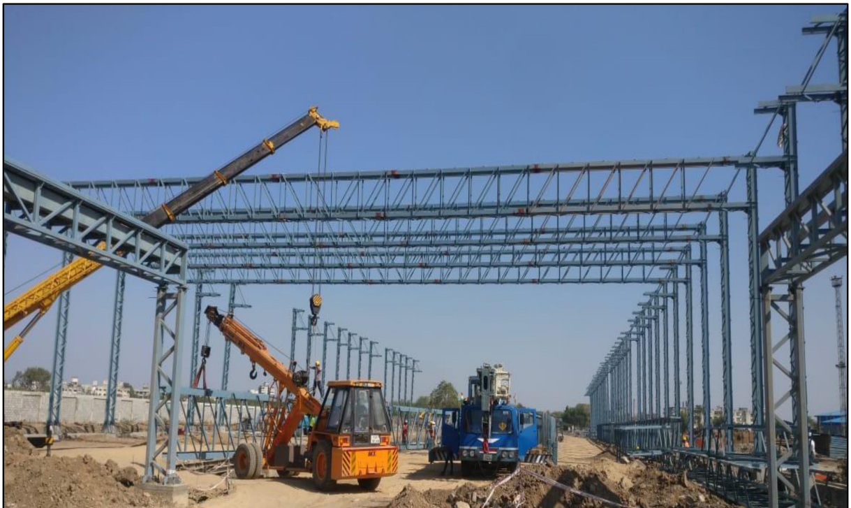
Gantry 1 – Beam under erection at Flash Butt Welding Workshop, Ahmedabad, Gujarat
