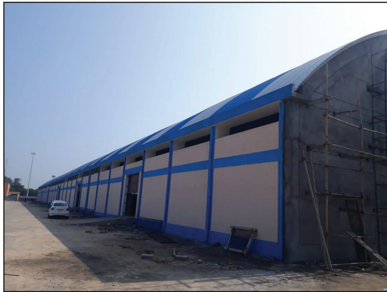
External Finishing Works in progress at CONCOR Khodiyar Warehouse 2, Sabarmati, Gujarat
