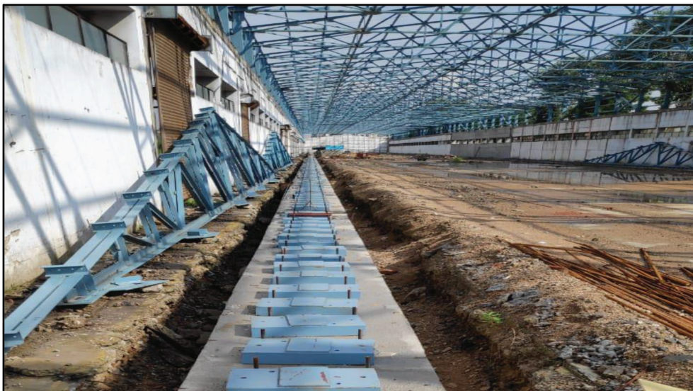
Goliath Foundation Works at Bridge Workshop, Sabarmati, Gujarat
