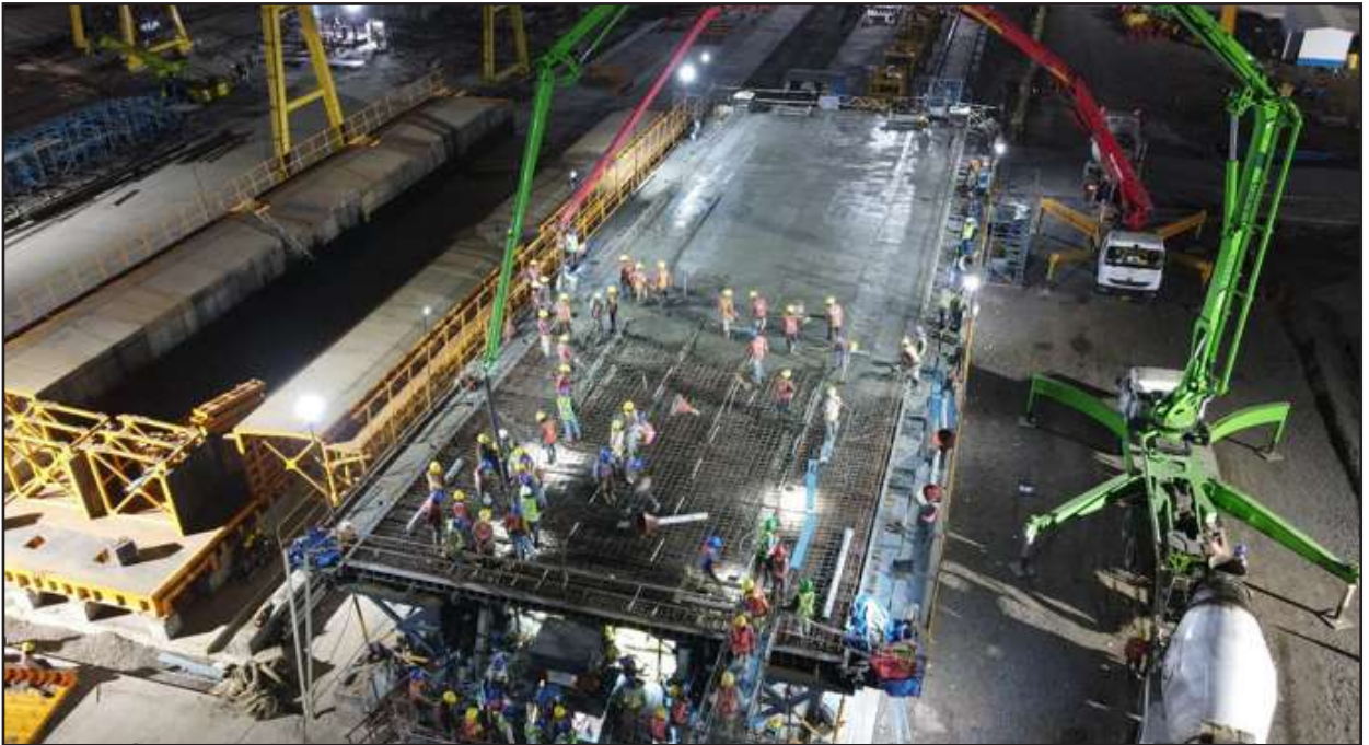
Full Span girder casting in progress, Anand, Gujarat
