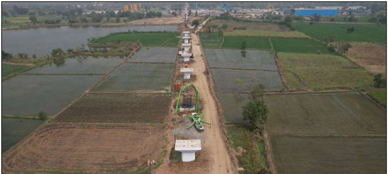
Pier work in progress, Billimora, Gujarat
