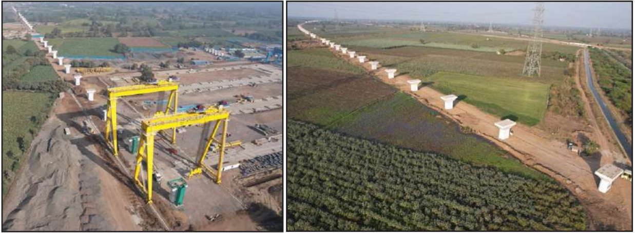
Completion of Pier & Pier cap works, Gujarat
