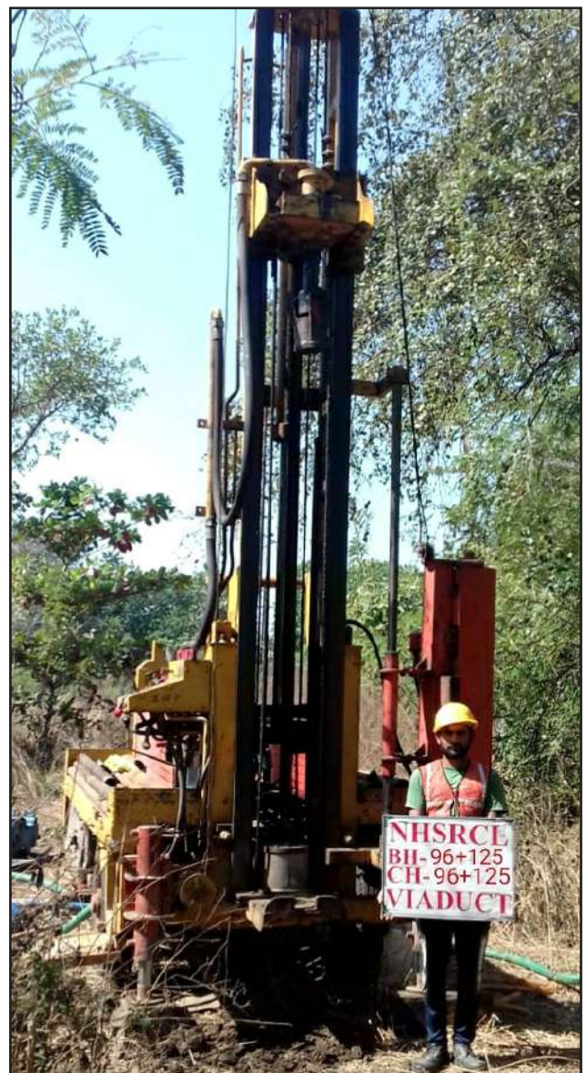
Geo-Technical works, Palghar, Maharashtra
