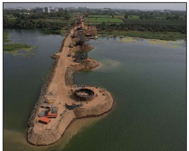
Well foundation work in progress at Tapi River, Surat, Gujarat
