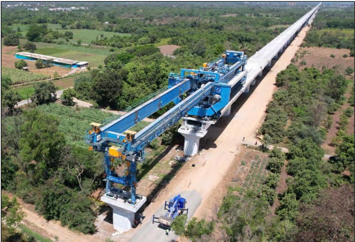
*Full span girder launching in progress, Navsari, Gujarat*
