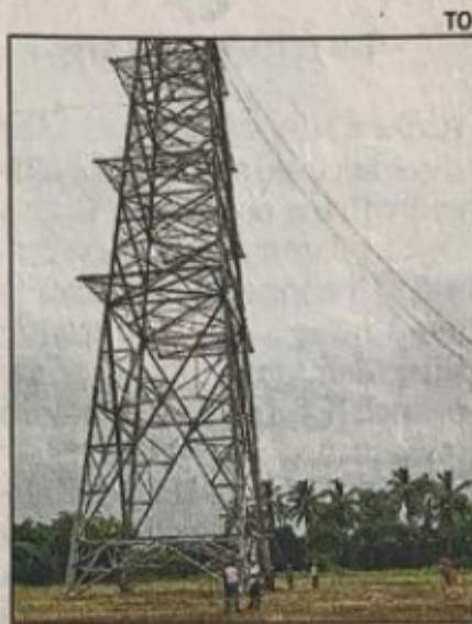
NHSRCL is relocating more than 1,600 electrical lines
