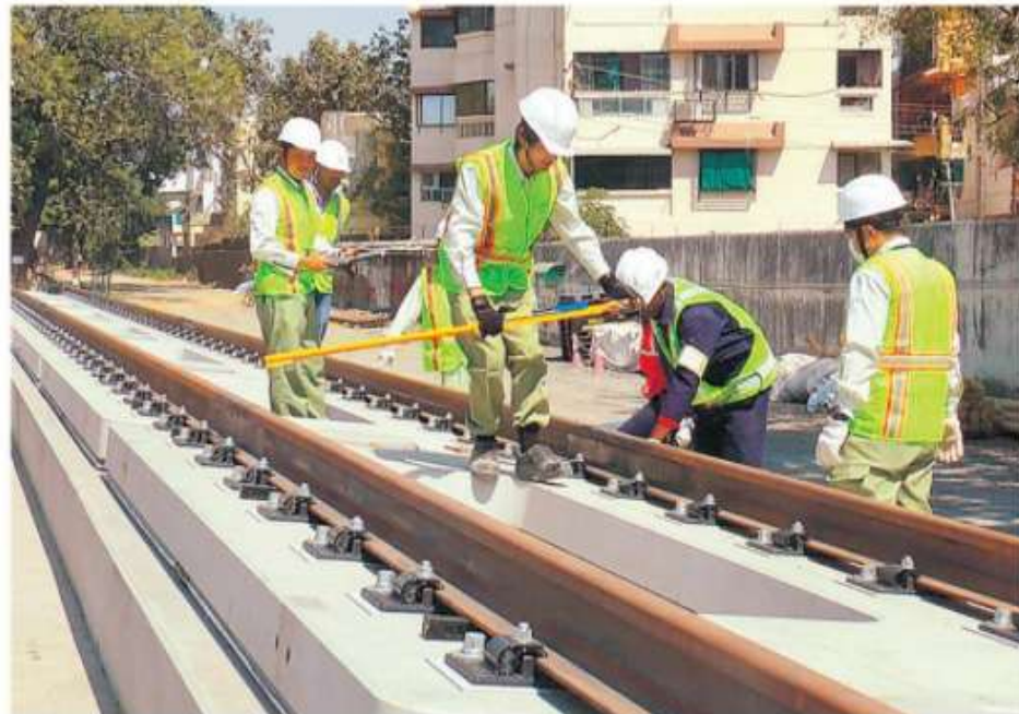
A template of the bullet train track being prepared at Vadodara
