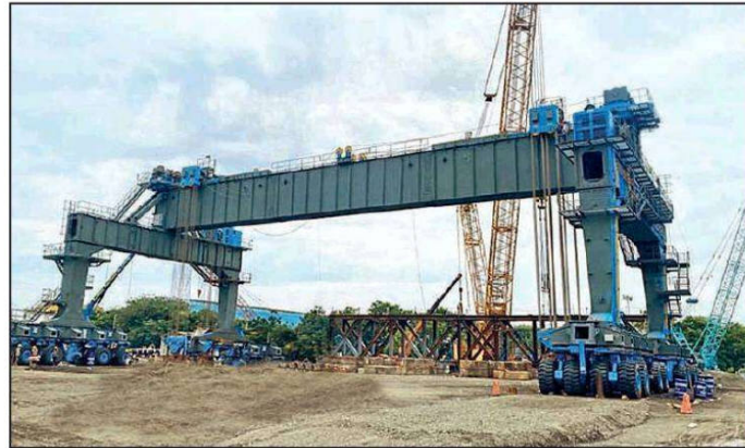
A straddle carrier and girder transporter
