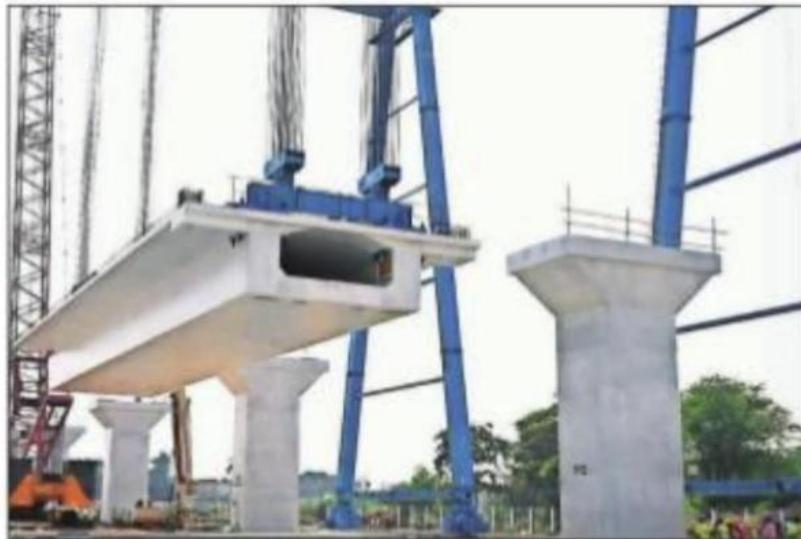
The girder consists of 390 cubic metres of concrete and 42 MT of steel and has been cast in a single piece. *Express*
