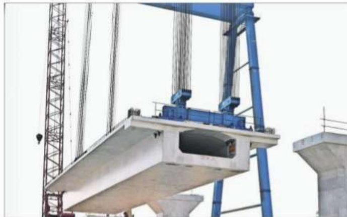
First girder erection at Navsari in Gujarat on November 25, 2021
