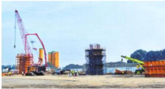
Girders and pillars being cast at the yard
