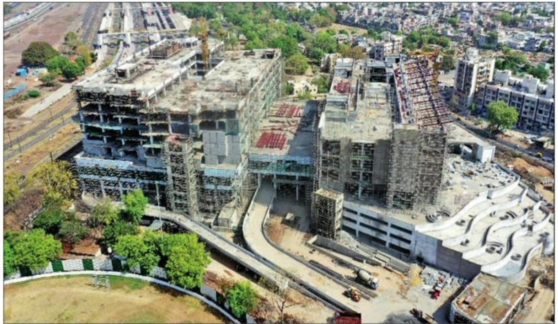
The passenger terminal hub under construction at Sabarmati railway station. (Right) Construction underway of a bridge over Sabarmati river
