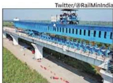
A bullet train girder being launched earlier this week
