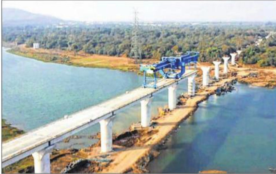
Construction of the first river bridge of the Mumbai-Ahmedabad High Speed Rail Corridor over Par River in Valsad is in full swing.
