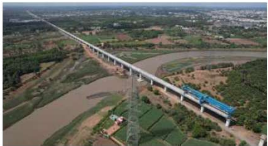
Picking up pace: The Purna river bridge is the second of the bridges to be completed as part of the project. SPECIAL ARRANGEMENT
