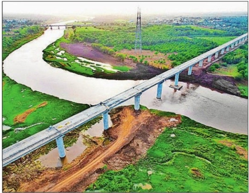
The longest bridge is 360 metre-long over Purna river in Navsari
