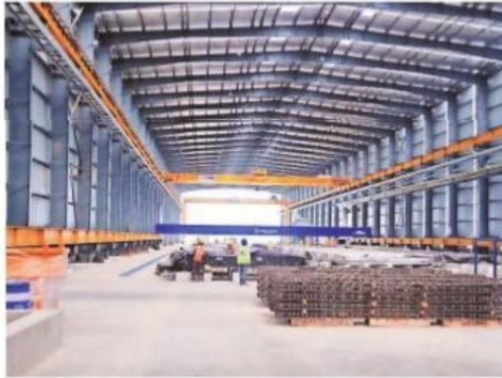
The Track Slab Manufacturing Facility is fully automated. Express
