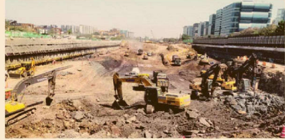
Excavation at Bandra Kurla Complex, where the underground Mumbai station of Mumbai-Ahmedabad high-speed rail is being built
