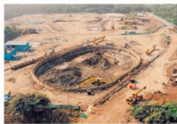
Work underway at Shilphata, Vikhroli and Sawli
