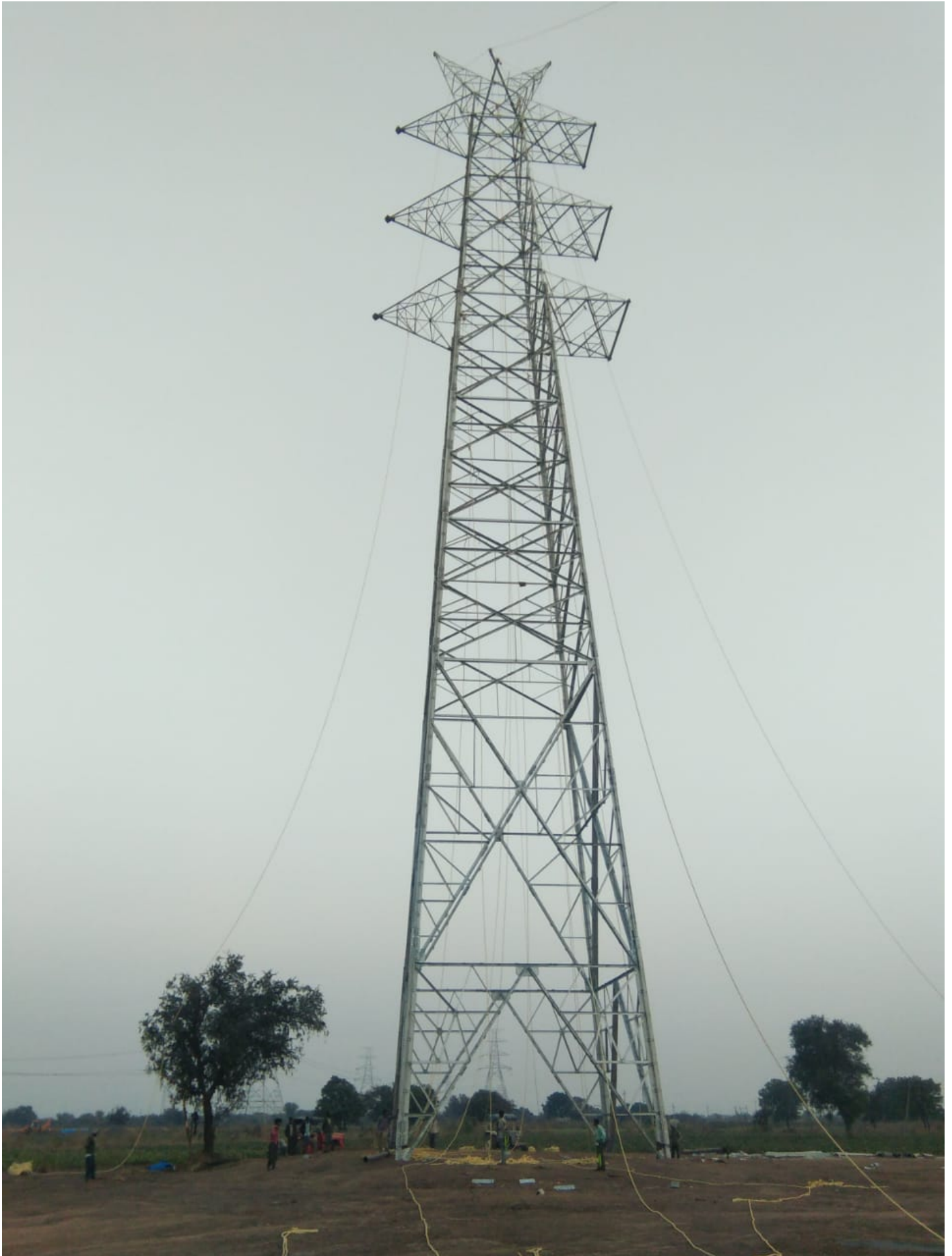
Images: Relocation work of 66 kV extra high tension line in Surat area
