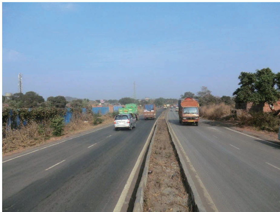
Figure 5.1.3: Road conditions in the vicinity between the SGNP and TWLS
