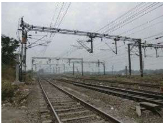
Figure 4.7-19 Existing Railway Line Near Proposed HSR Station
