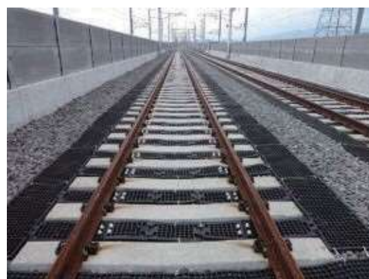
Figure 4.6-18 Ballast Track (installed with ballast screens)
