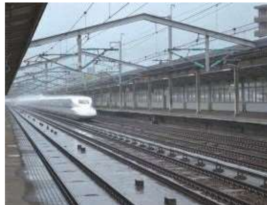
Figure 4.6-21 Slab Tracks of San-yo Shinkansen
