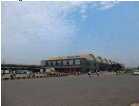
Figure 4.7-5 Lokmanya Station Building
