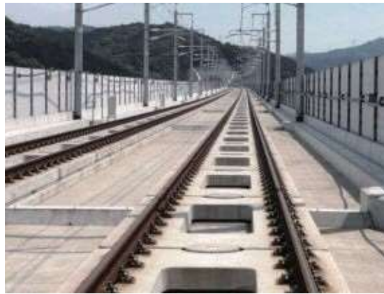
Figure 4.6-22 Frame-type Slab Track
