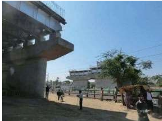
Figure 4.7-12 Road Over Bridge above the Existing Railway Line (Under Construction)
