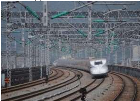
Figure 4.6-20 Ballast Tracks of San-yo Shinkansen
