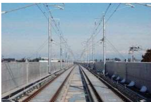
Figure 4.6-17 Plate-type Slab Track
