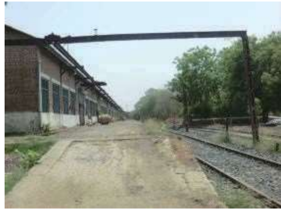
Figure 4.7-92 Warehouse for Rail Welding
